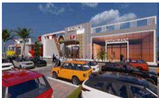
THE LEGACY MALL, DODOMA Works Ongoing
